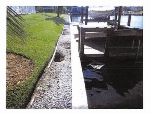
Symptoms: Sinkholes upland of the wall, visible back-fill mounds in the water near bulkhead joints (most visible at low tide).
