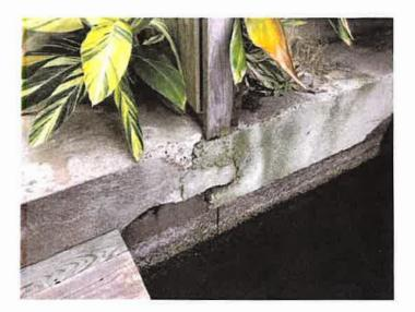
**Symptoms:** The principal symptoms are rust, spalling, exposed rebar, and fractures.
